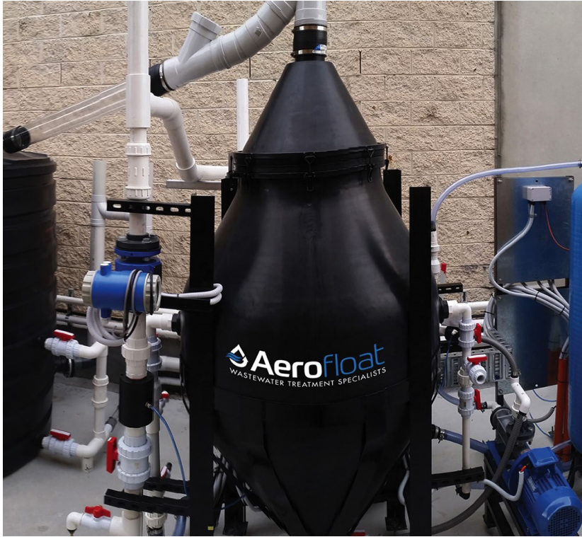
LEFT: Aerofloat's patented world-first technology Dissolved Air Flotation (DAF) technology is compact, affordable, low maintenance, odourless and self-cleaning.
