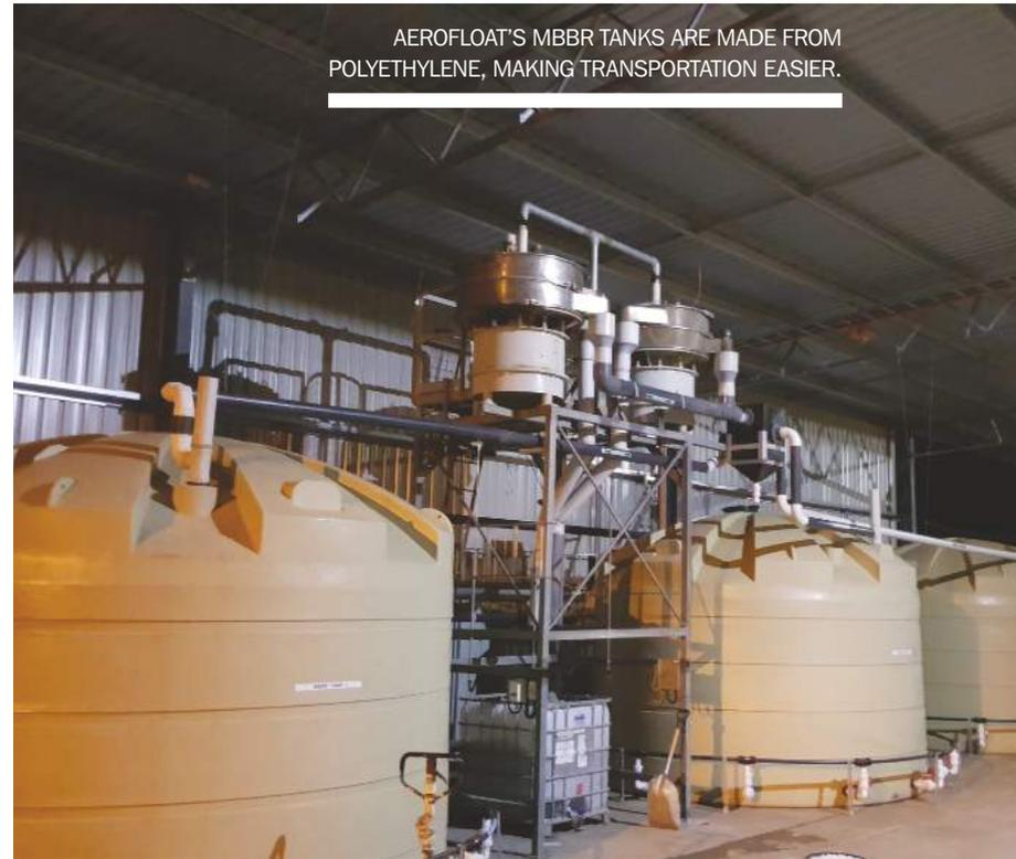
AEROFLOAT'S MBBR TANKS ARE MADE FROM POLYETHYLENE, MAKING TRANSPORTATION EASIER.
