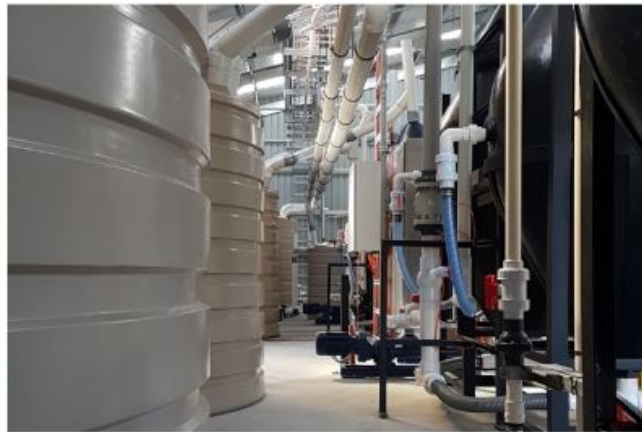
ABOVE: The implementation of Dissolved Air Flotation (DAF) and Moving Bed Biofilm Reactor (MBBR) technology from Aerofloat is underway.
